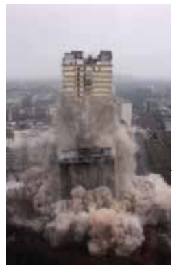
Sprengung des AfE-Turms, 2. Februar 2014 \ Blowing up the AfE-Turm, February 2, 2014 \ © Foto photo: Boris Zdravkovski
